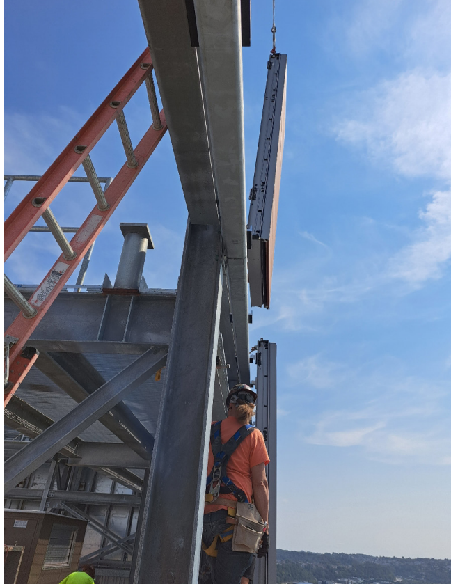
A member of Ironworkers Local 3 working on construction. Credit: Marshall Long
