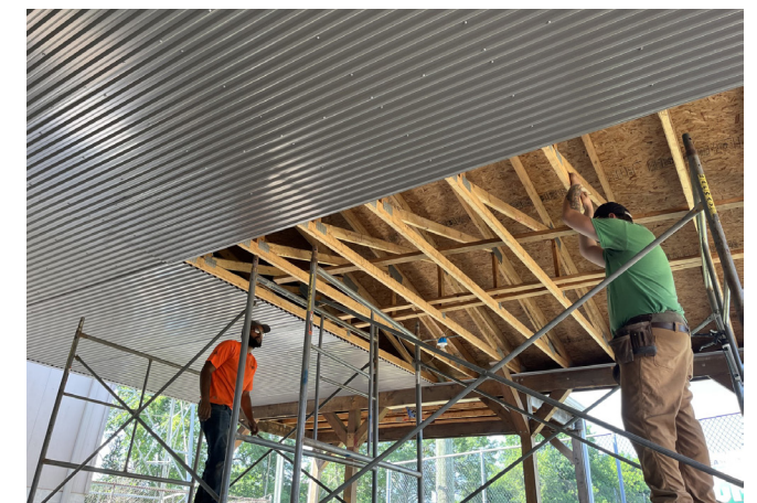
Pennsylvania union members on a construction job
