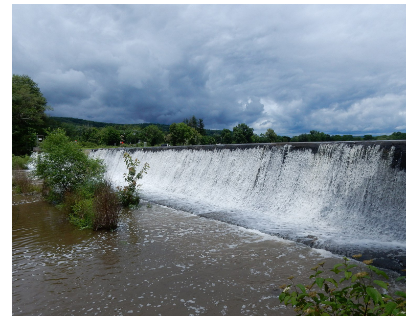
Deer Lake Dam in Schuylkill County
